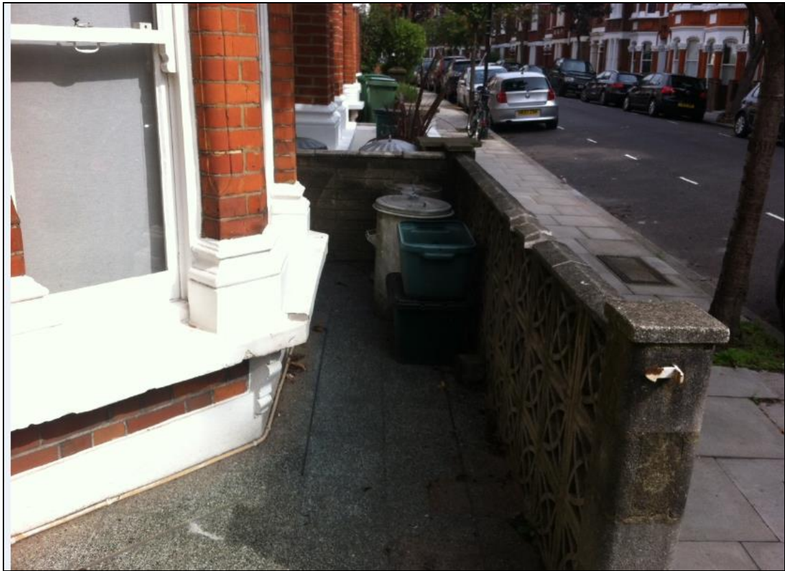
Photo 4: Existing front boundary wall and tiling
