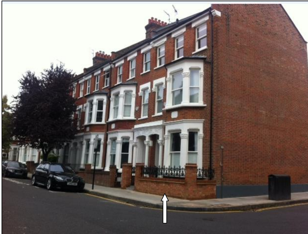
Photo 5: Corner property No.55 Calabria Road which received planning permission P122193 and has constructed front lightwell with new boundary frontage.
